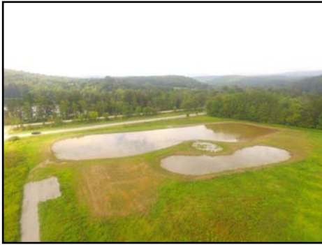
Newly constructed wetland after a heavy rain. Drone photo courtesy of Patrick Repko.
